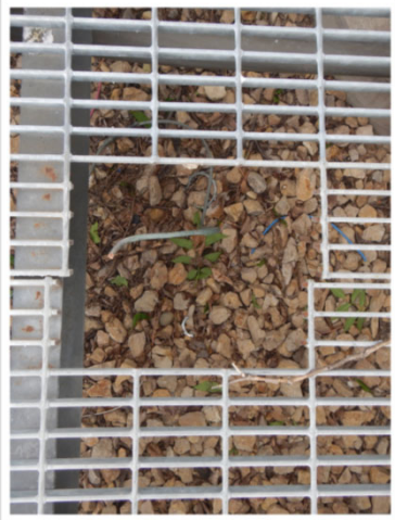
Hole in Platform
